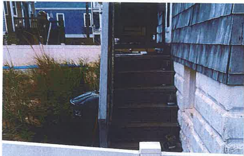
#60 First Ave - East Door
